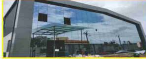
Glazing, ACP, 12 mm Skylight
