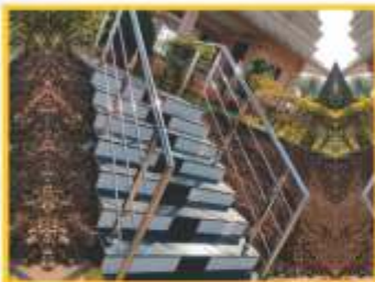
S.S. Pipe Railing
