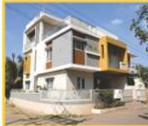
Glass Railing, Windows, Skylight
