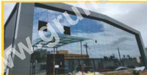
Glazing, ACP, 12 mm Skylight
