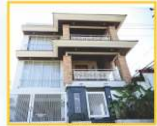
Windows, Skylight, Glazing
