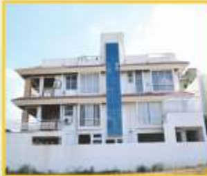
Windows, Skylight, Glazing
